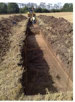
boreholes, cone penetration testing and trial pits. Samples were taken to assess geotechnical properties of the soils. Geophysicl analysis included thermal resistivity of the soils and seismic refraction/ reflection to determine the underlying geology of the salt marsh which was inaccessible to plant. Utilities surveys were also carried out at each of the proposed crossings.
