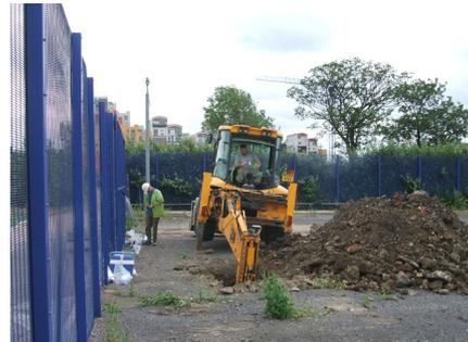
The site works proved challenging as shallow obstructions from previous structures and foundations were encountered.
