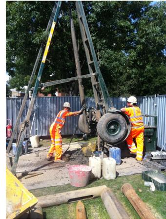
Drilling locations were generally situated within parks and on highways and pavements, where public access required secure compounds to be set up, often within areas underlain by numerous underground services requiring service tracing and clearance systems to ensure safe working practices. All excavations and subsequent reinstatement works were supervised and undertaken by appropriately trained NWRSA-qualified operatives & supervisors.
