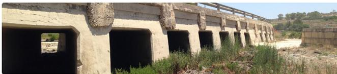
The original road was built on a concrete walled embankment sitting on a shallow concrete foundation, including numerous culverts to allow water to flow to the sea during heavy rainfall. Transport Malta's original plan was to widen the road by building the two additional lanes on rock fill embankments and elevated concrete structures founded on bearing piles. During tendering, contractor KOSTA joint venture proposed a more cost-effective alternative, replacing the piles with a floating raft.
