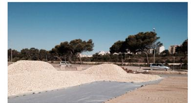
This separator layer prevented differential settlement of the compacted rock embankment fill and provided additional structural stiffness. The embankments were built up in stages to pavement level and the final surface laid, once settlements had reduced to acceptable levels.
