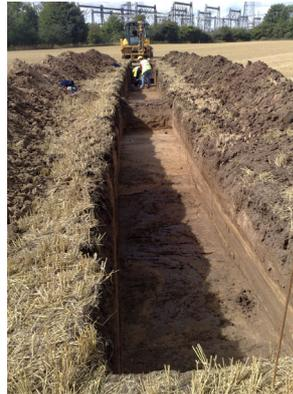
boreholes, cone penetration testing and trial pits. Samples were taken to assess geotechnical properties of the soils. Geophysical analysis included thermal resistivity of the soils and seismic refraction/reflection to determine the underlying geology of the salt marsh which was inaccessible to plant. Utilities surveys were also carried out at each of the proposed crossings.
