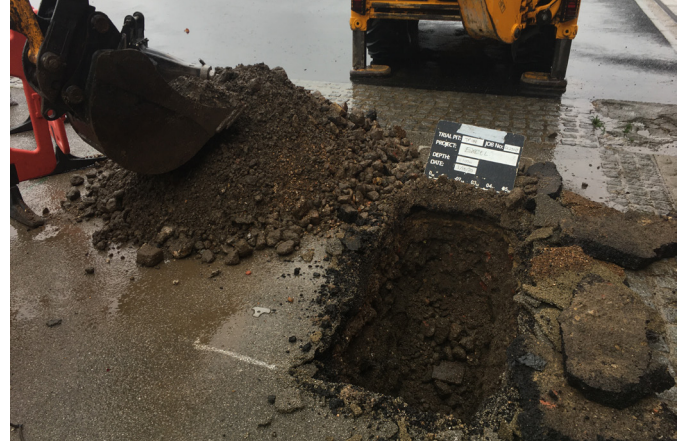
Typical machine-excavated trial pit
