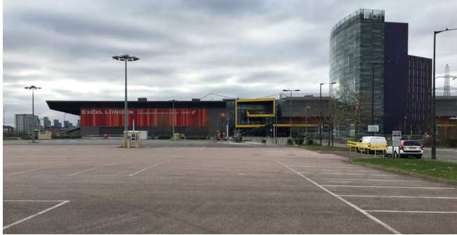
ExCel Exhibition Centre & eastern car park
