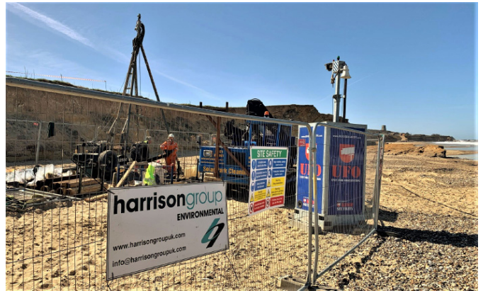
Site compound for the drilling work
