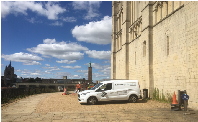
Site work at the castle overlooking Norwich
